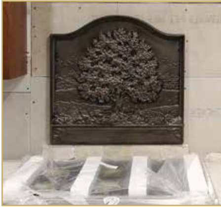
Fireback glued or mounted to the hardie board
