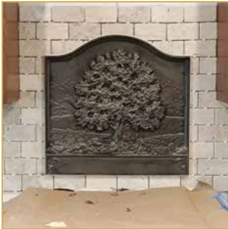
Tile placed around fireback after mounting
